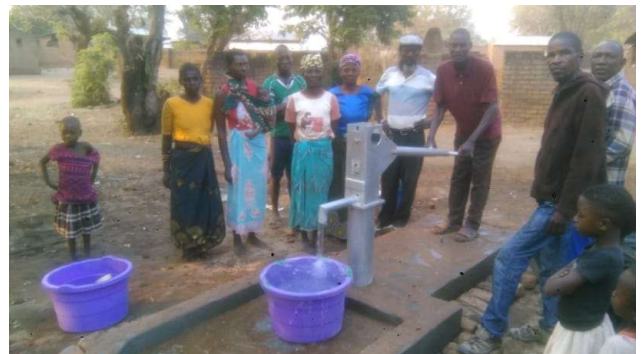
The completed borehole at Nsanje
