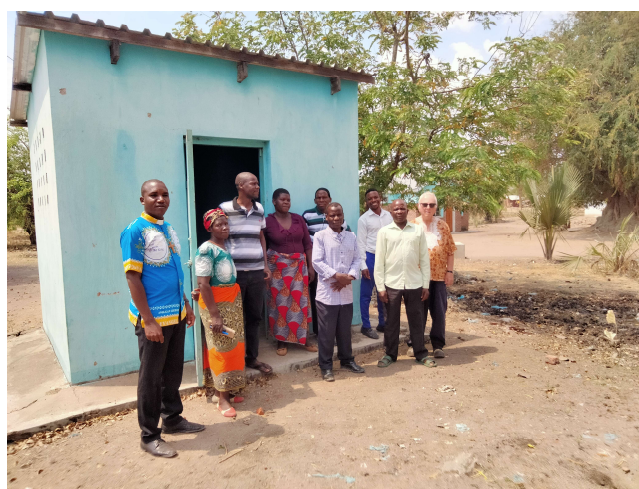
The Lundu Health Committee outside the Solar Pump Control Hut.
