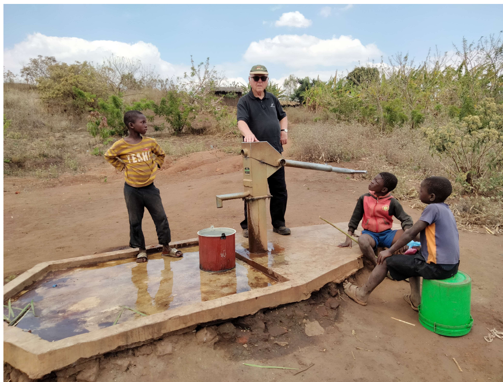
The Njuli rehabilitated pump
