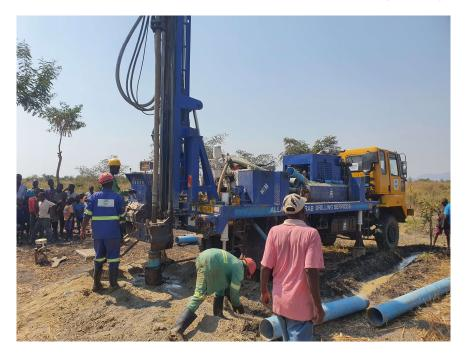
Left- Drilling in progress at Lundu for the installation of the new pump
