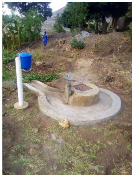
The second RORA donated borehole after refurbishment
