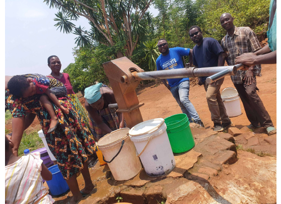
Rehabilitation of an Afridev borehole damaged by the cyclones
