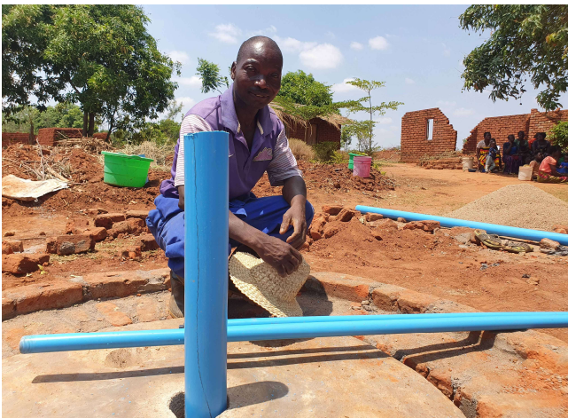
The pump liner being installed in the new borehole
