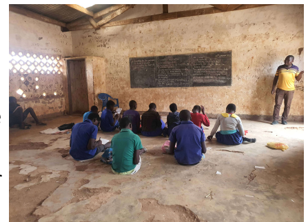
Classroom before rehabilitation
