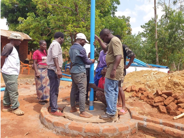
The pump liner being installed in the new borehole
