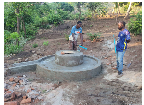
The above borehole refurbished
