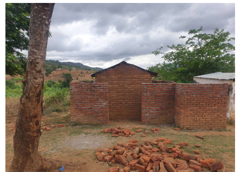
Girls toilet after refurbishment
