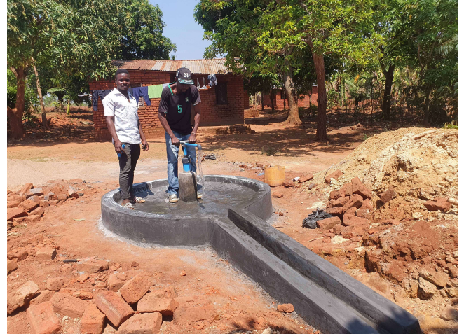
The first completed borehole at Mulanje
