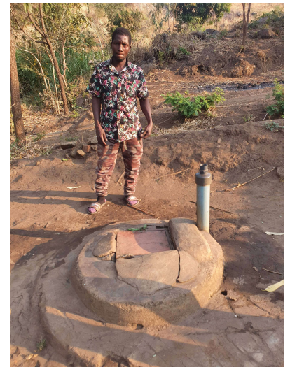
One of the RORA donated boreholes before refurbishment
